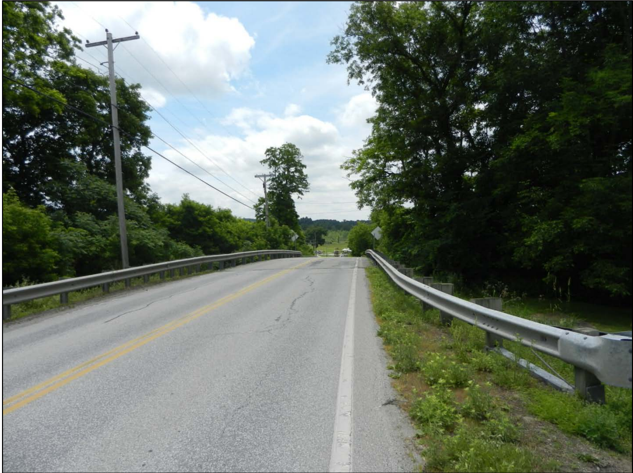
Figure 2 Photograph of bridge as viewed looking south.
