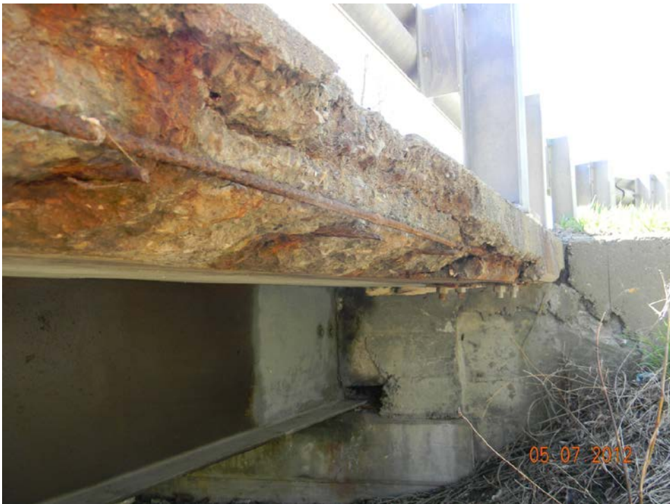
Close-up, west side of bridge deck looking south
