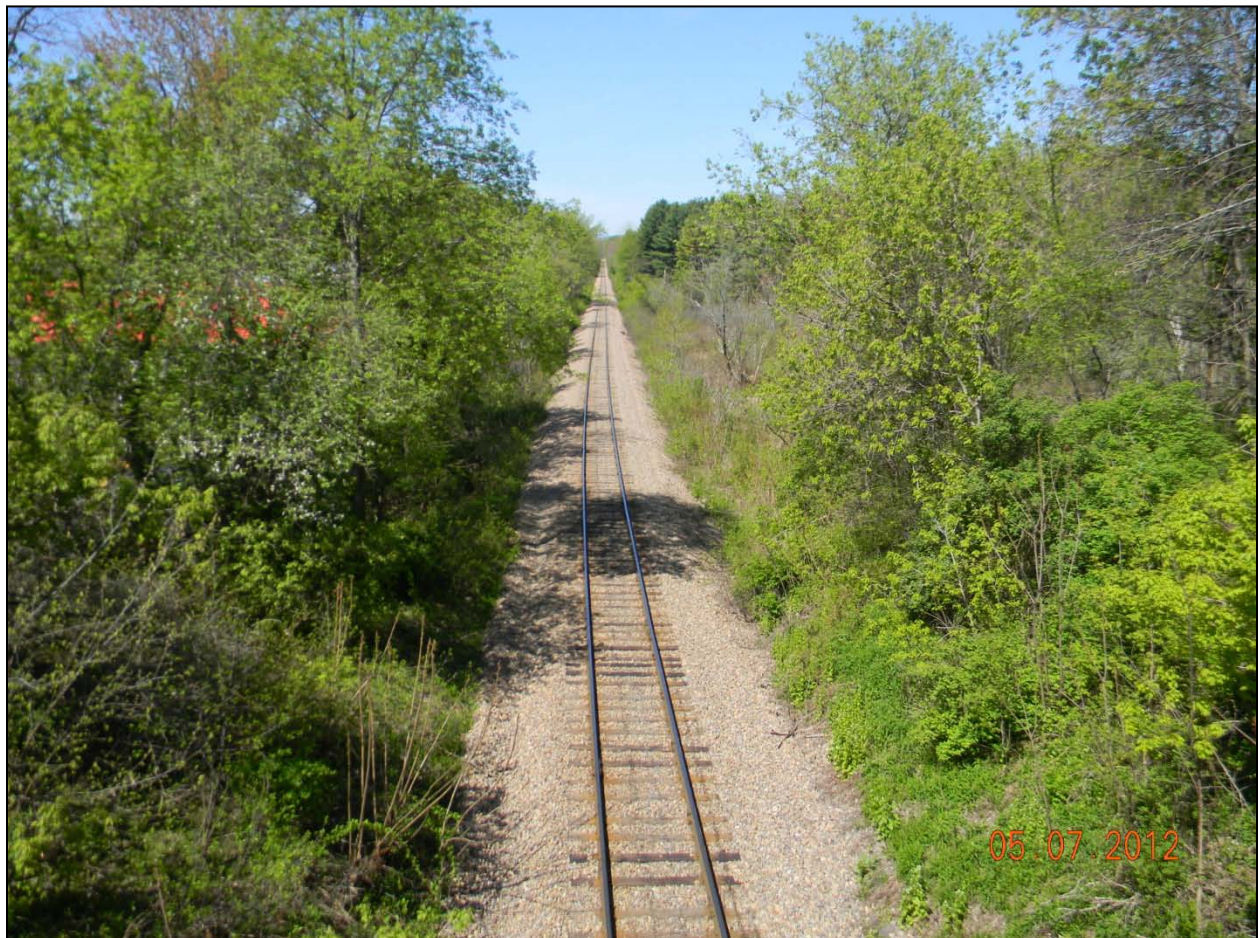
Figure 1 View of railroad grade at Bridge 93.
