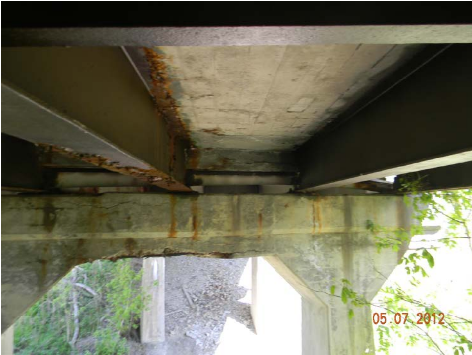
Underside of bridge looking north
